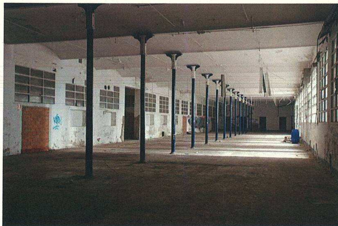
Interior de la nau de can Carbonell i Reveter
